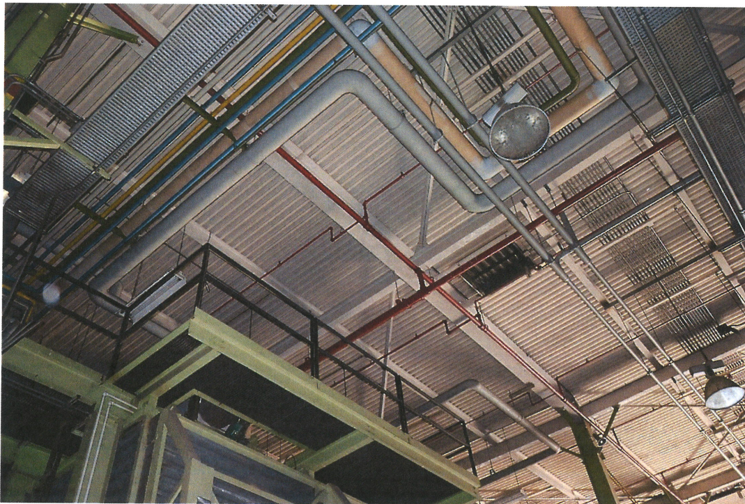
Roof in West building addition
