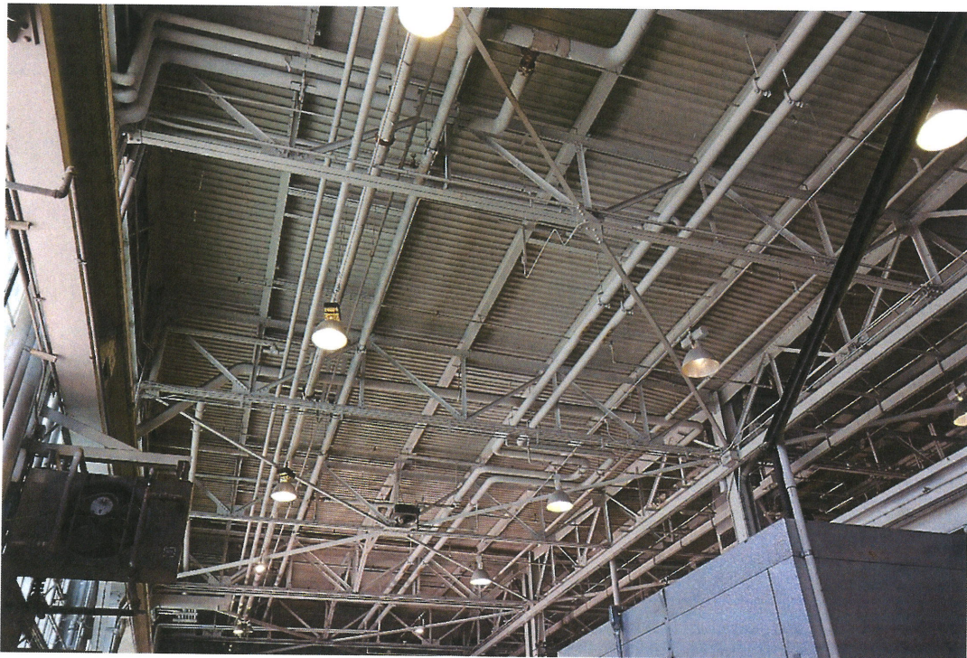
Roof above Shop Area
