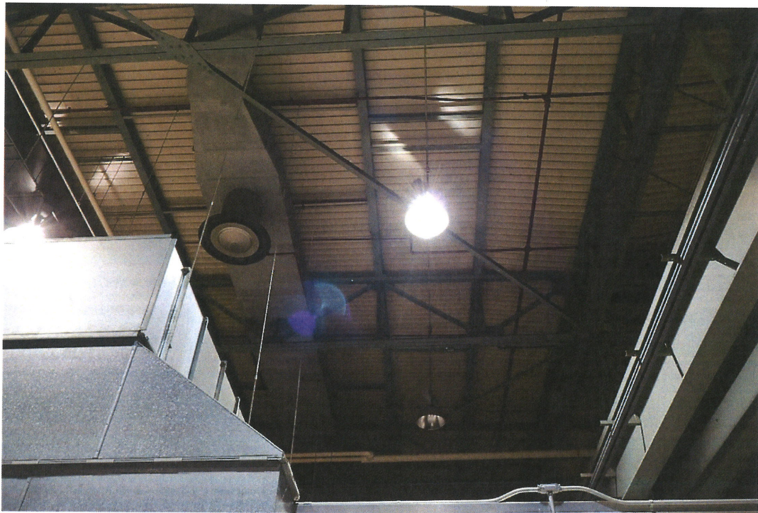
Roof in Retubing Area
