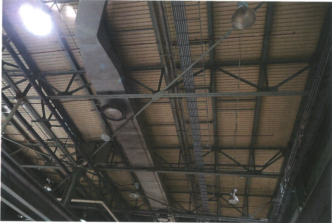
Roof in Retubing Area
