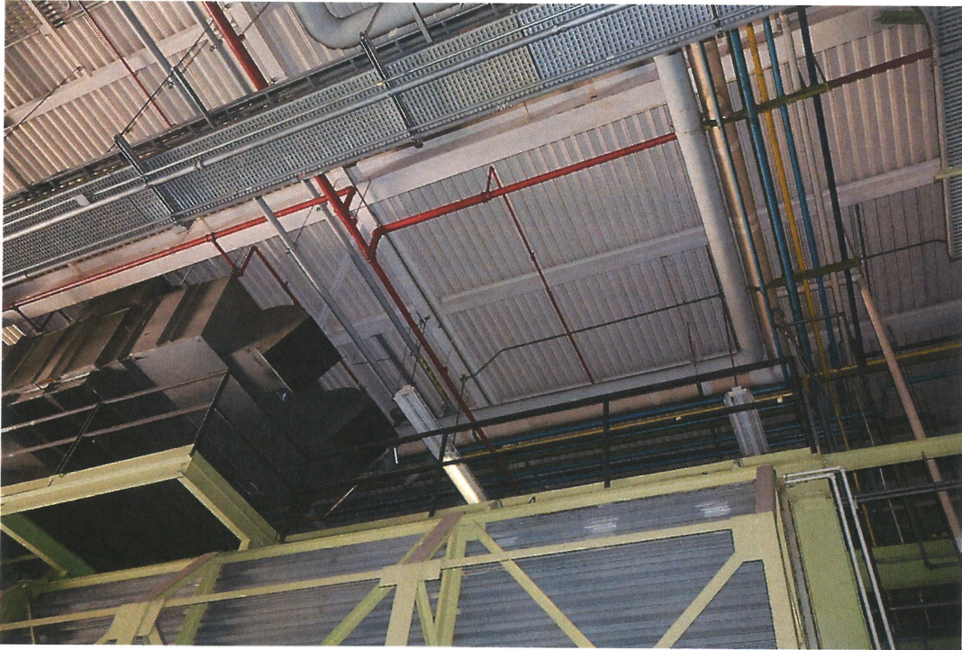
Roof in West building addition
