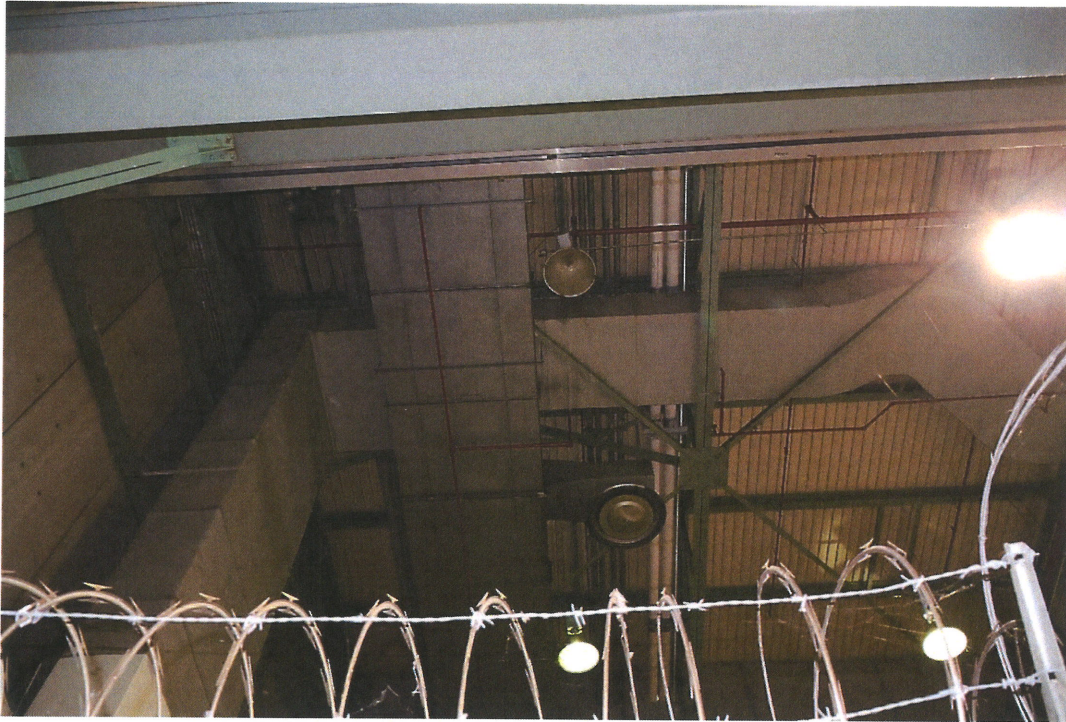
Roof on Northeast side of Retubing Area
