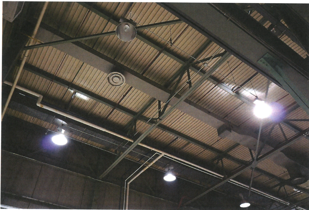
Roof in Retubing Area
