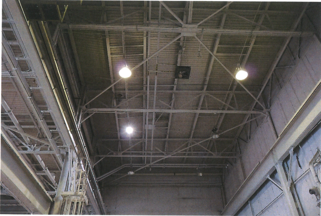
Roof on Northeast side of Shop Area
