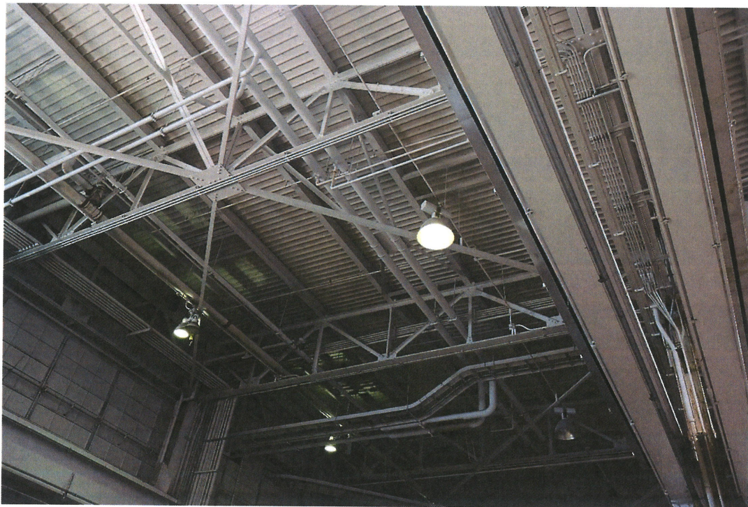
Roof on Northwest side of Shop Area
