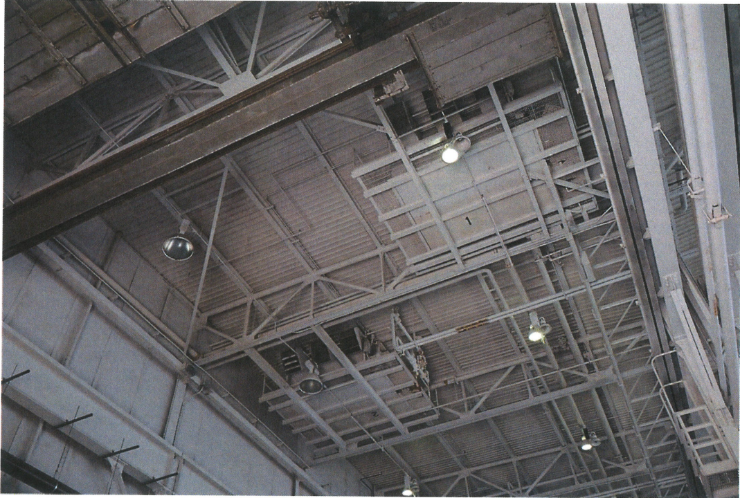
Southeast corner of building
