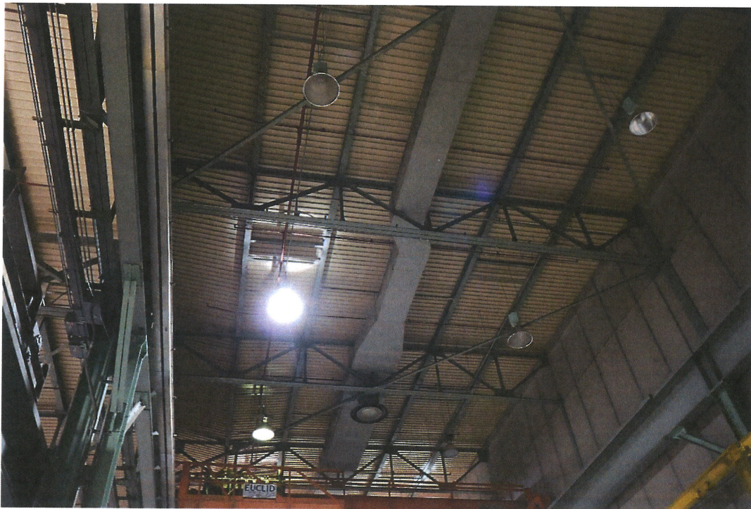
Roof in Retubing Area
