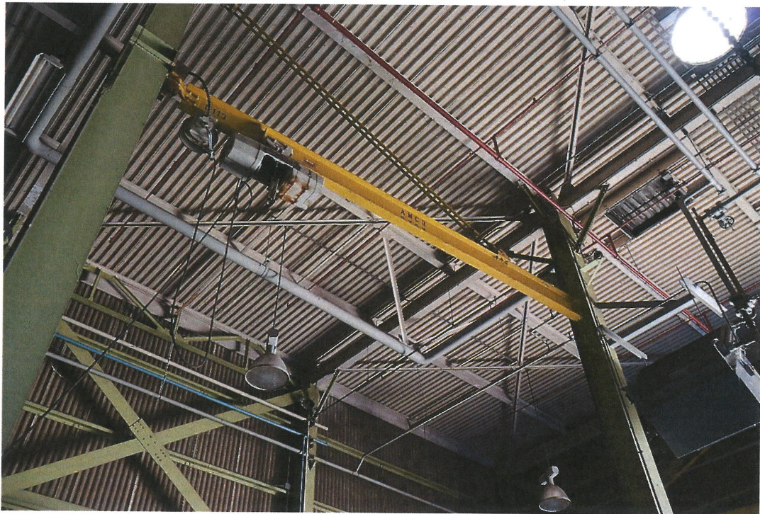
Roof in West building addition
