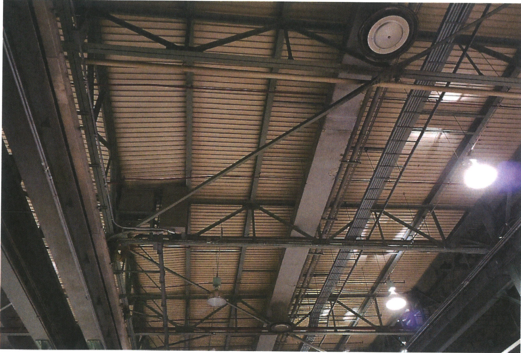
Roof in Retubing Area
